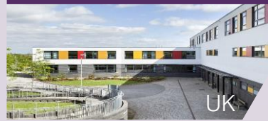
Sheffield Student Accommodation
